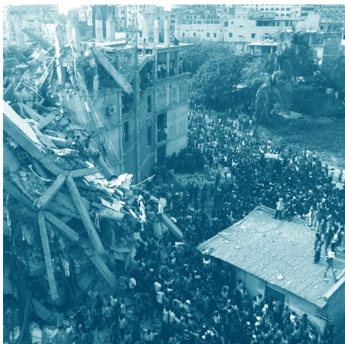
Fabrik Rana Plaza/Foto Int. CCC
